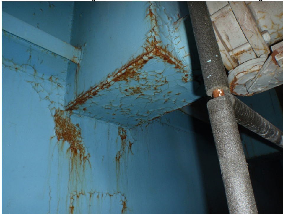
Pictures 14: Rust on the exterior of filter along welds on inlet box and interior backwash trough.
