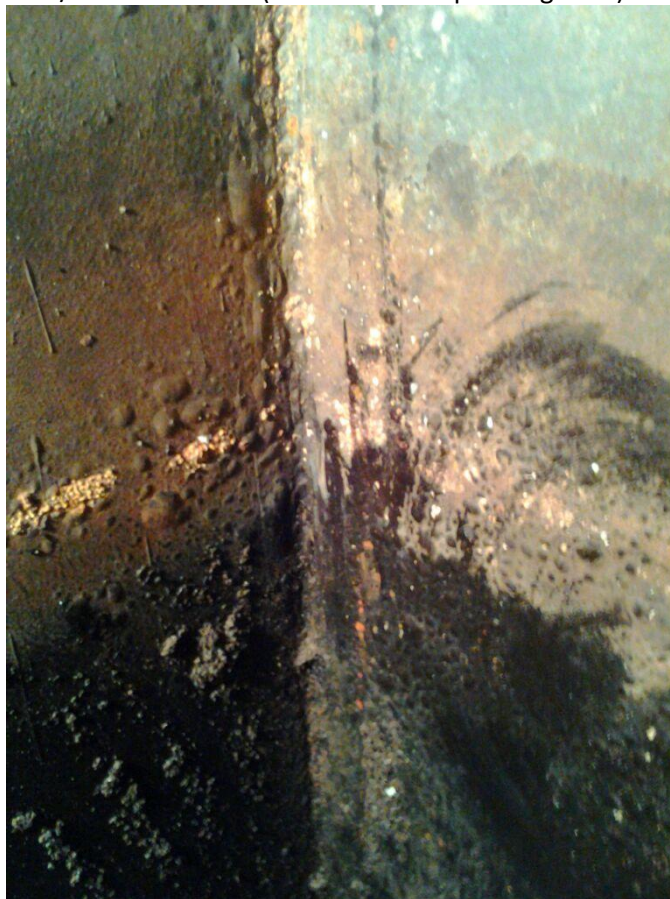
Picture 21: Corner of filter bed at air/water interface (normal water operating level).
