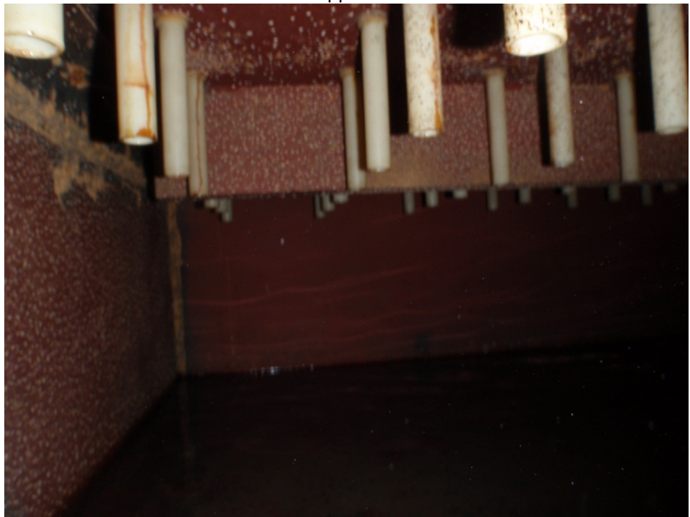
Picture 3: Filter distributors and structural elements appear to be intact. Minor rust can be seen in corner welds.
