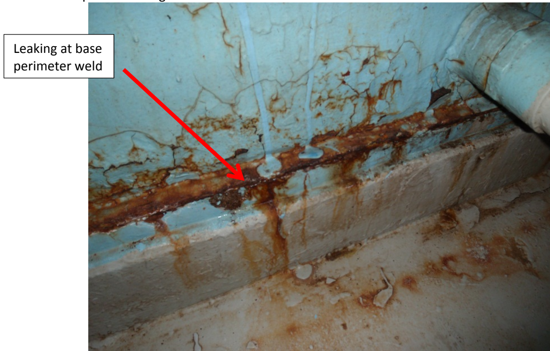
Picture 12: Close up of rust along west side filter base.
