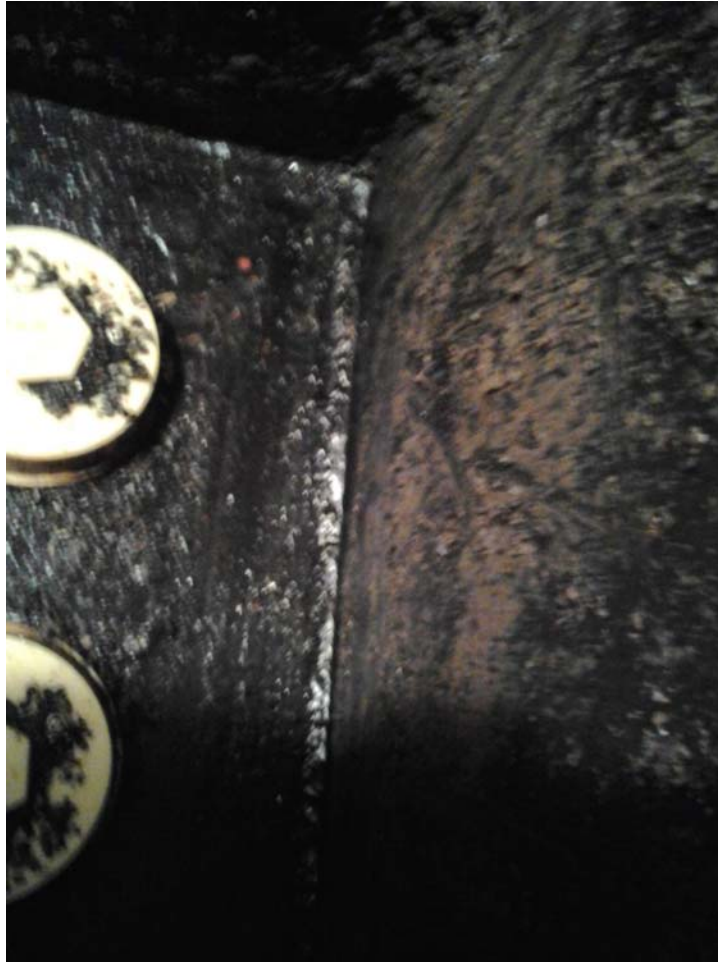
Picture 23: Close up of filter bed base and wall joint. No apparent rust and paint appears to be intact.
