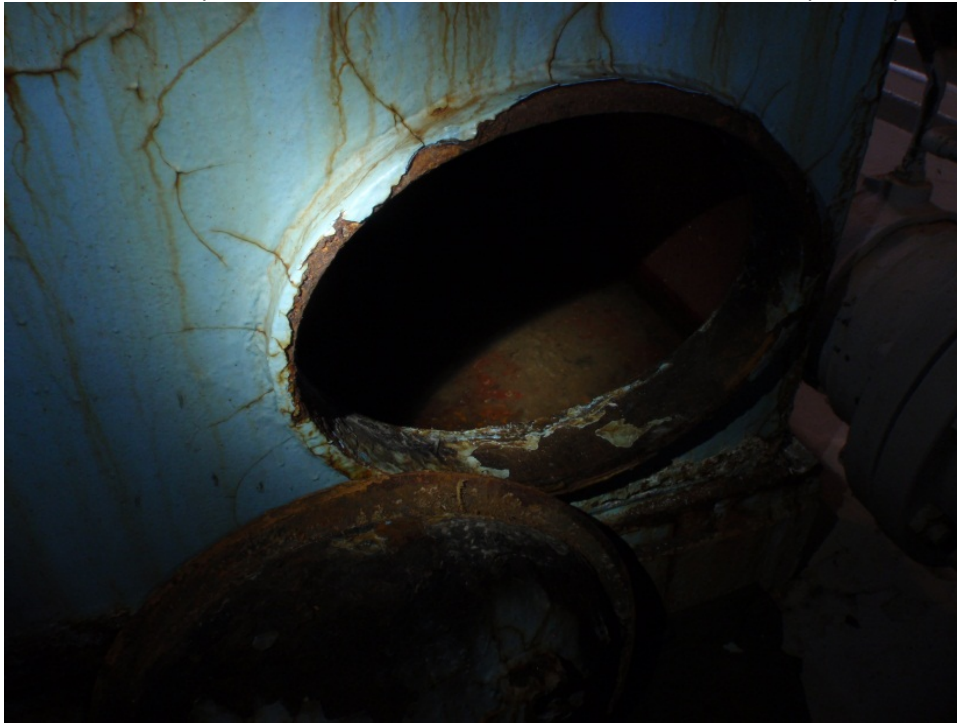
Picture 7: Apparent rust deteriorating the interior of the manhole
