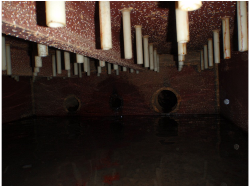
Picture 4: Far end of underdrain; backwash, effluent, and air scour piping. Leaking can be seen in center air scour piping.
