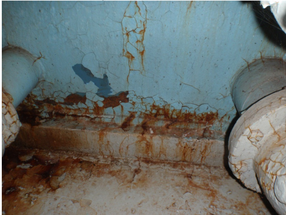
Picture 10: Rust can be seen at the base of the filter in the pipe gallery on the east side of the filter. Piping makes accessing the exterior filter base difficult.
