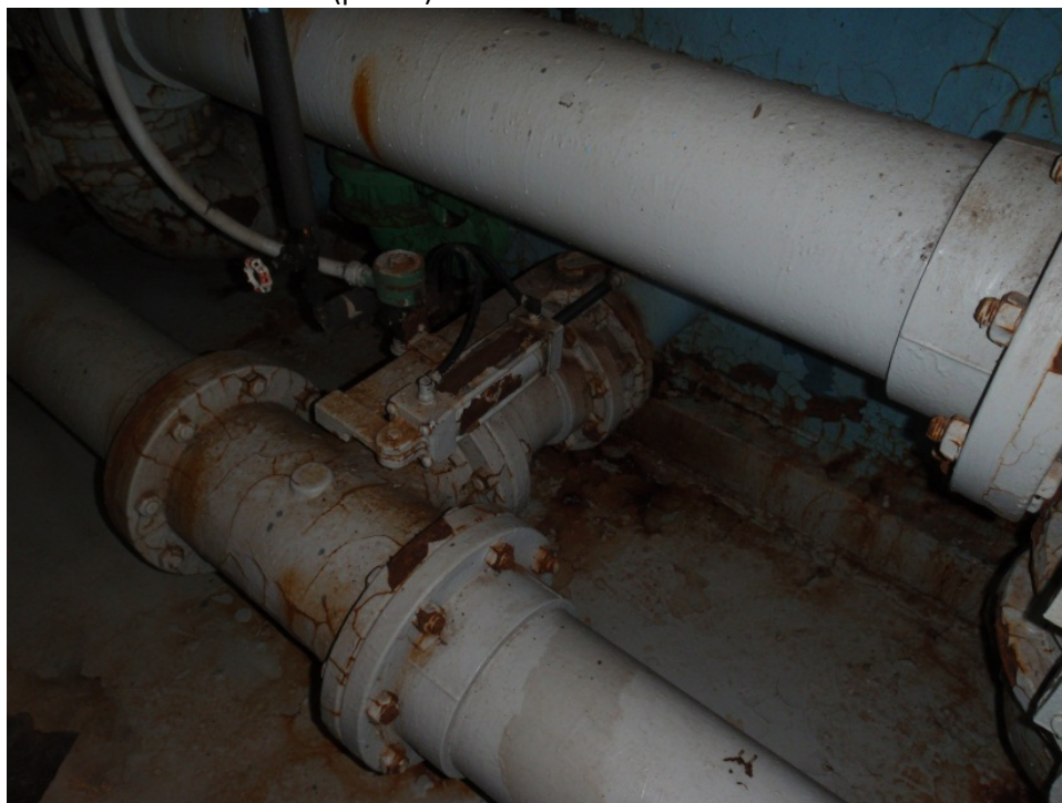
Picture 19: Rusting valve and valve actuator (piston).
