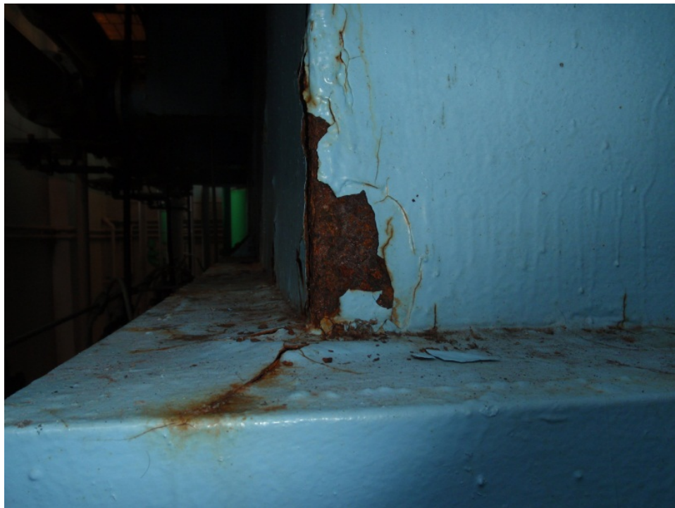
Picture 16: Rust on the northeast corner of the filter above horizontal structural member.
