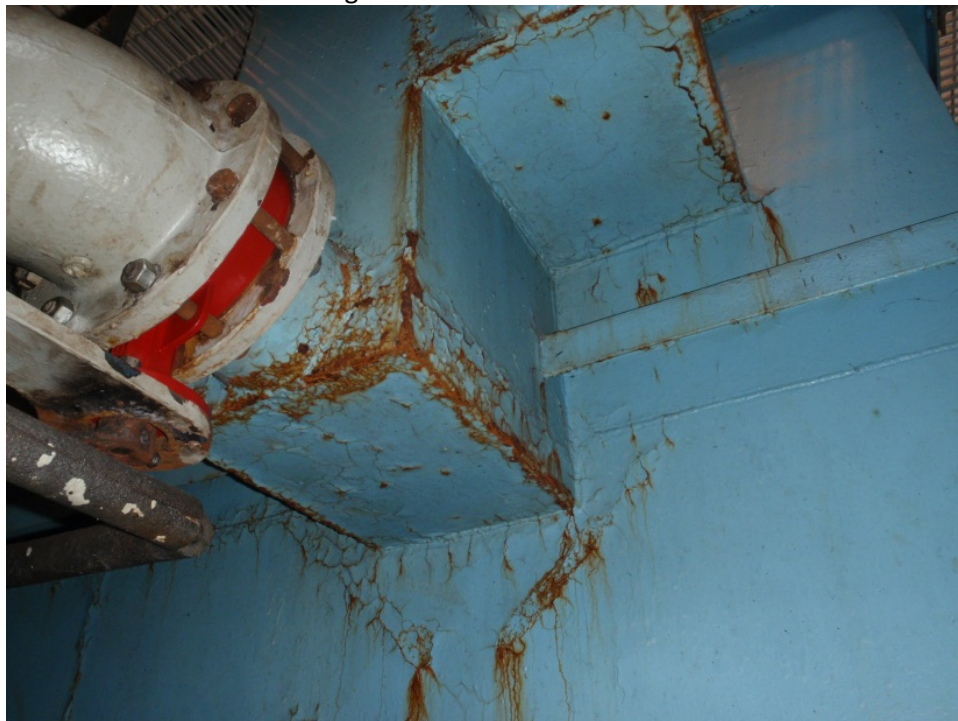
Picture 15: Rust on the exterior of the filter along welds on the inlet box.
