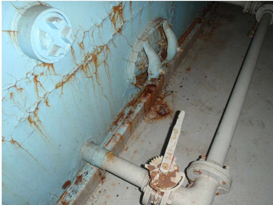
Picture 11: Rust can be seen at the base of the filter in the on drain side (west). Rust has caused the most significant deterioration and leaking along the west filter base.
