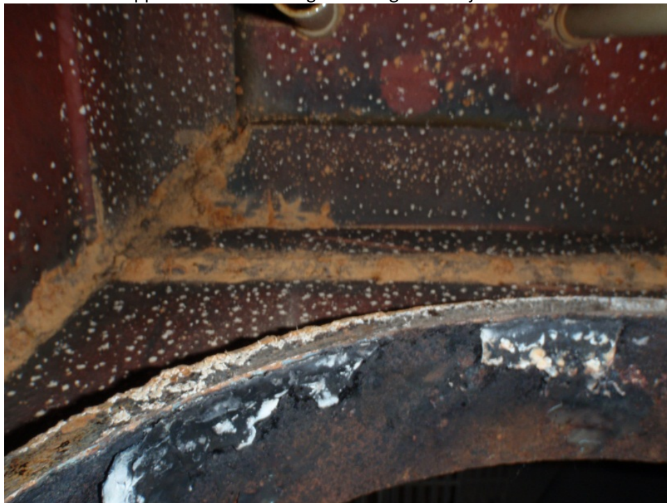
Picture 5: Apparent minor rusting occurring at weld joints in underdrain.
