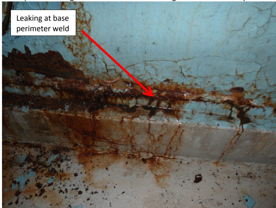
Picture 13: Second close up of rust along west side filter base. Leaking can be seen in this picture.
