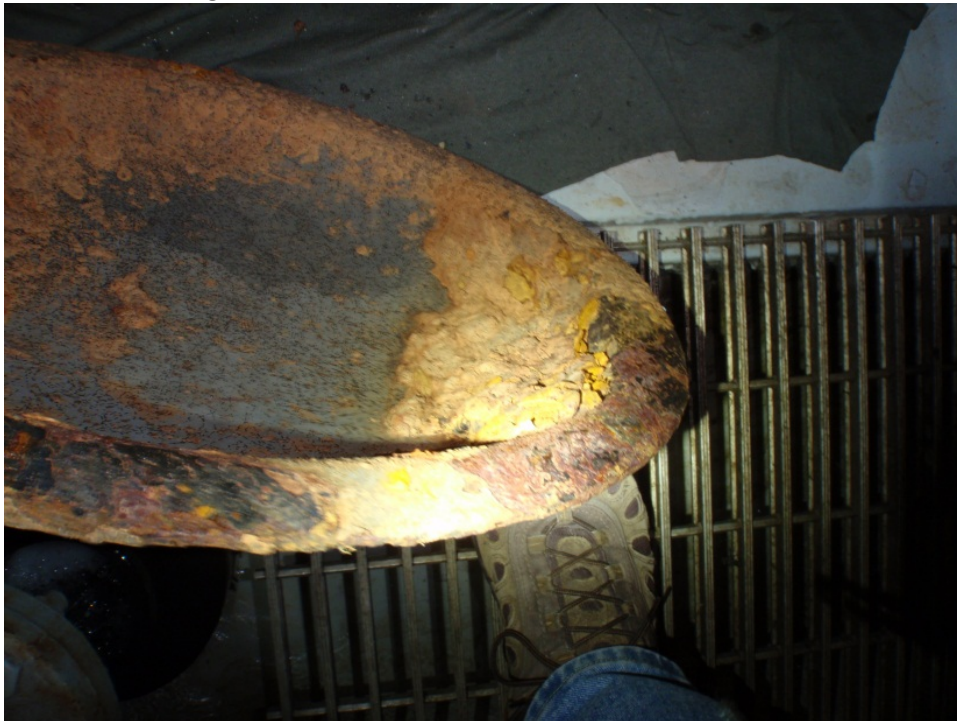
Picture 7: Apparent rust deteriorating the interior of the manhole
