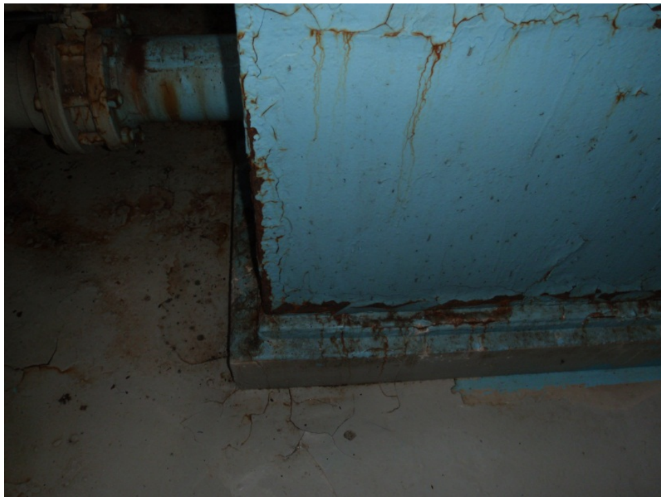
Picture 17: Rust on the northeast corner of the filter above the base.
