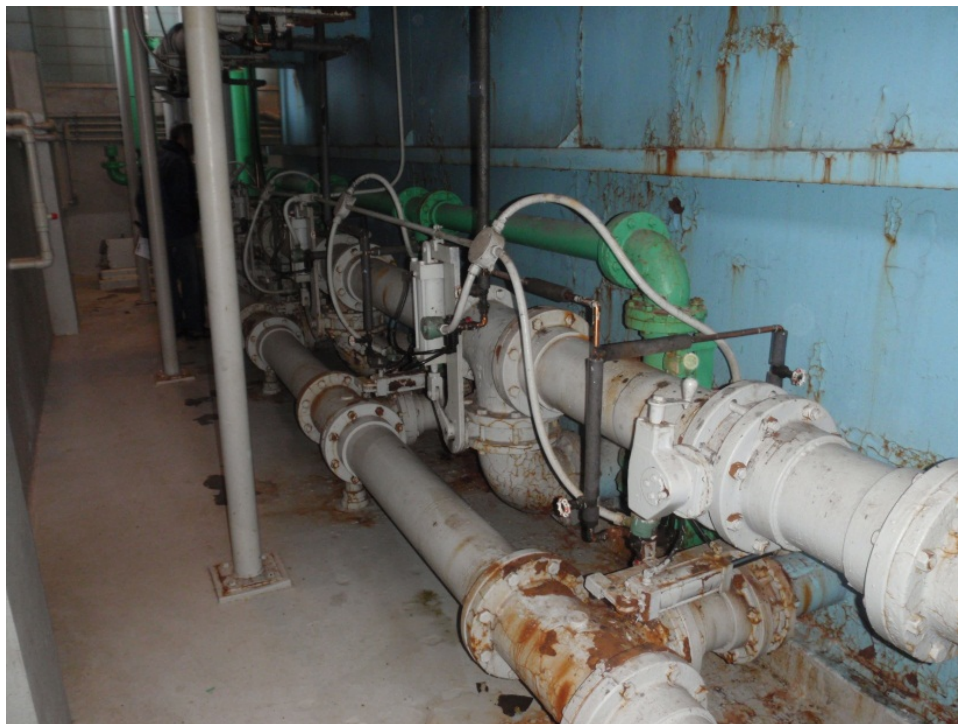
Picture 18: Pipe gallery along the east side of the filter. Rust can be seen on the exterior of the filter and cast iron tee fittings.
