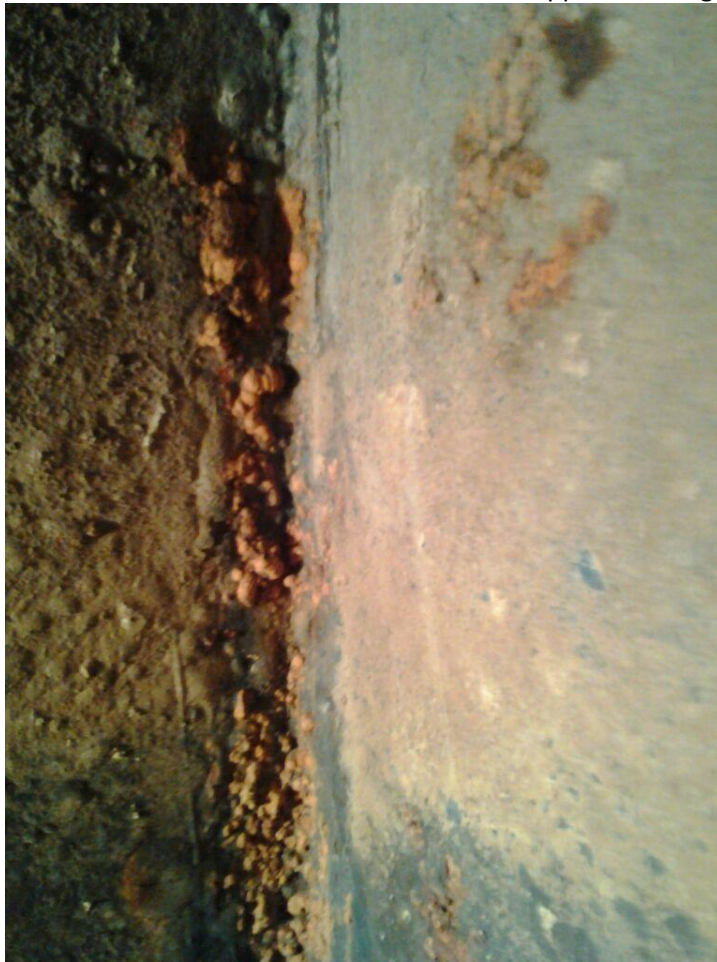
Picture 22: Close up of air/water interface on interior of filter. Minor rust apparent along welds.
